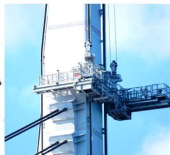
写真-1 塔外面作業車 Photo 1 Maintenance Gantry for Tower
