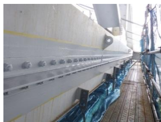
写真-1 トラス部材補強 Photo-1 Steel Truss Member
