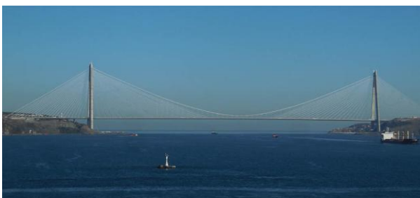
写真-3 橋梁全景 Photo-3 The 3rd Bosphorus Bridge
