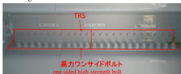
写真-2 当て板設置完了 Photo-2 Completion of plate splicing
