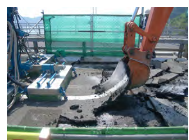
写真-3 既設舗装剥ぎ取り状況 (Photo.3 Removal of existing pavement)
