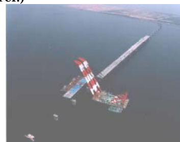
桁架設 (Installation of Girder)
