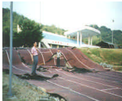
断層のずれ Slip of fault
