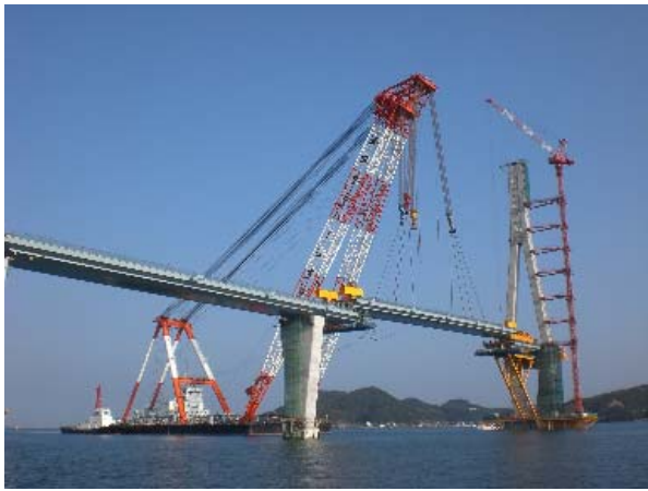
写真-6 側径間架設状況 (Photo.6 Construction of side span)
