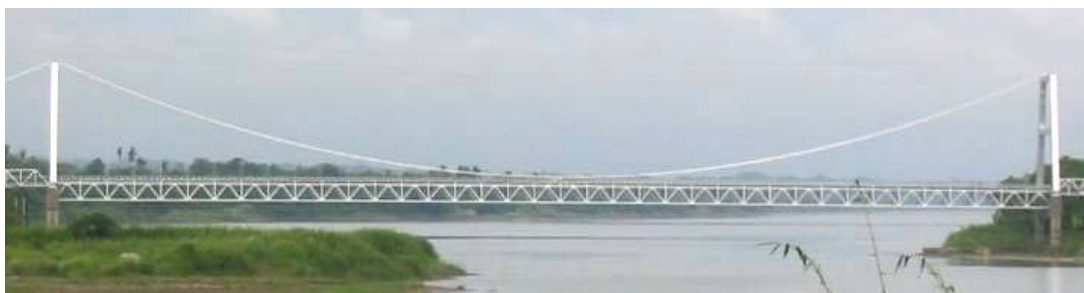
写真-2 マガピット吊橋全景 (Photo.2 Full View of the Magapit Suspension Bridge)
