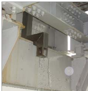
写真-1 排水樋 (Photo 1: Drain gutter)
