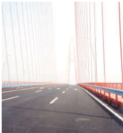
桁上より View from the deck
