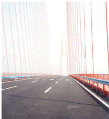
桁上より View from the deck
