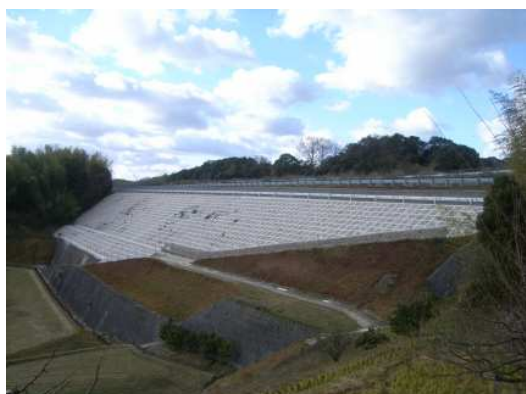
のり面防災対策
