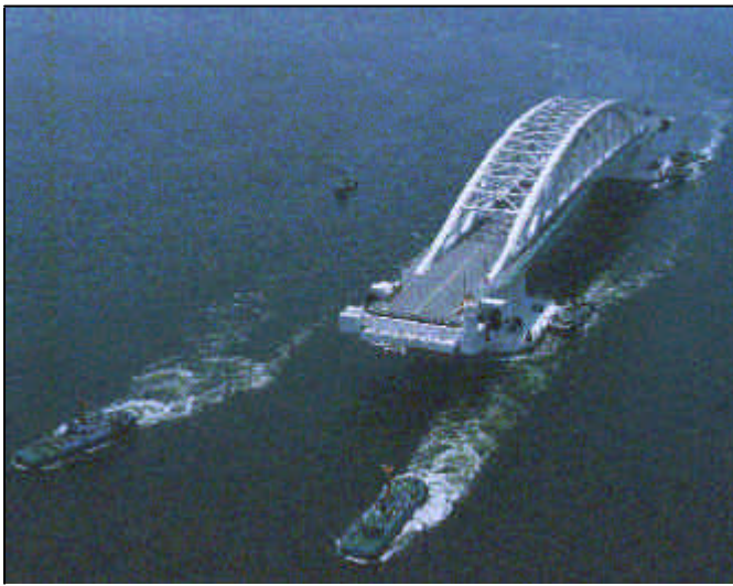
夢洲～舞洲連絡橋の曳航 Towing of Yumeshima-Maishima Bridge
