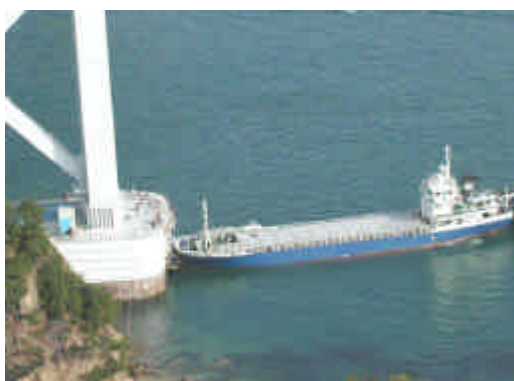
北備讃瀬戸大橋3Pへの船舶衝突 (Ship Collision against a Pier)
