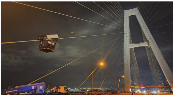
写真-7 施工状況 Photo 7 Repair Work Situation
