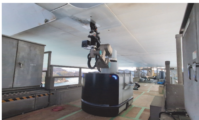
写真-3 補修塗装ロボットによる作業状況 Photo 3 Scenes of Work Performed by Repair Painting Robot
