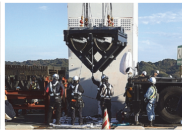
写真-2 5P 主塔部交換状況 Photo 2 Replacement near Main Tower (5P)
