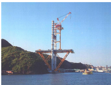
上部工架設状況 (Installation of superstructure)
