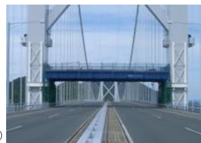
写真-3 路面防護工 (Photo.3 Protection for road )
