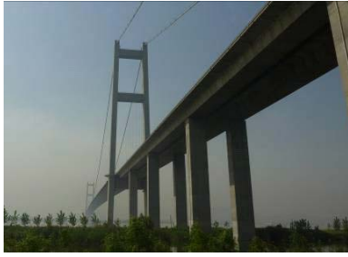
写真-6 潤揚大橋(吊橋) (Photo-6 Runyang Bridge) (suspension bridge portion)
