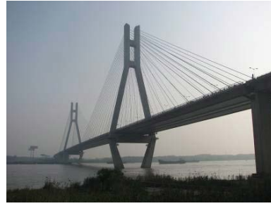
写真-7 潤揚大橋(斜張橋) (Photo-7 Runyang Bridge) (cable stayed bridge portion)
