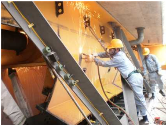
写真-5 損傷桁切断 Photo.5 Cutting damaged girder
