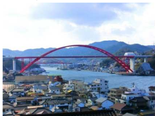
写真-4 第二音戸大橋全景 Photo.4 Over View of the 2 nd Ondo Bridge
