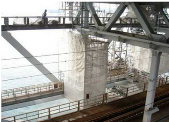
写真-1 仮設足場(枠組み足場) Photo-1 Temporary Scaffolding (Steel frame scaffolding)
