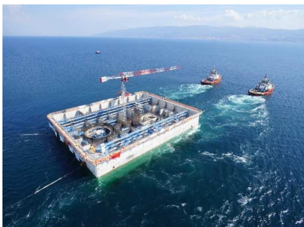
写真-6 ケーソンの曳航 Photo.6 Launching of Caisson Base
