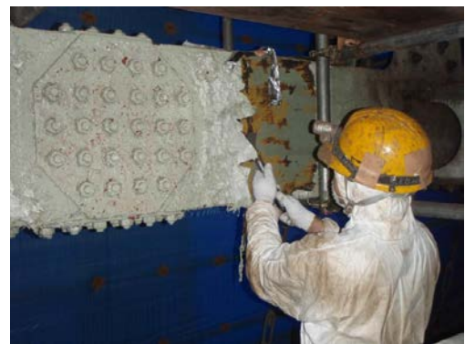
写真-4 塗膜除去作業 Photo.4 Paint removing work
