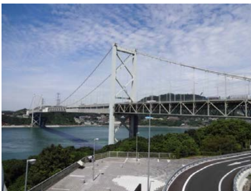
写真-3 関門橋全景 Photo.3 View of the Kanmon Bridge
