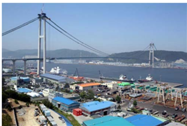
写真-5 補剛桁架設後の全景 Photo.5 View after erection of girder
