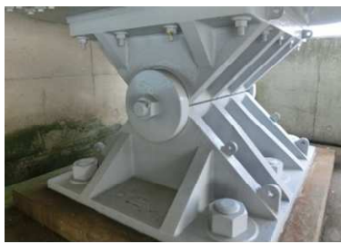
写真-1 トラス桁支承(交換前)・HVa30P Photo 1 Truss Girder Bearing Before Replacing (HVa30P)
