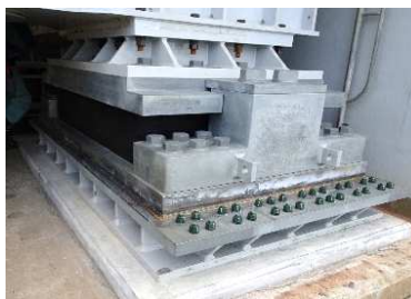
写真-3 トラス桁支承(交換後)・HVa30P Photo 3 Truss Girder Bearing After Replacing (HVa30P)
