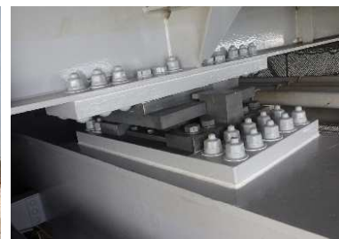
写真-4 道路桁支承(交換後)・SW1 Photo 4 Road Deck Bearing After Replacing (SW1)
