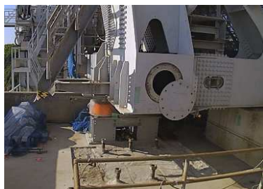
写真-2 トラス桁支承(交換中)・HB1P Photo 2 Truss Girder Bearing in Replacing (HB1P)
