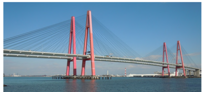
写真-6 名港西大橋全景（写真奥：I期線、手前：II期線） Photo-6 Meiko Nishi Bridges (Front: westbound bridge, Back: eastbound bridge)
