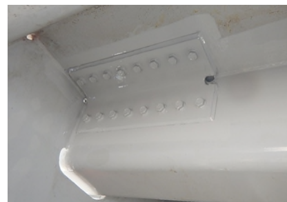
写真-4 施工完了 Photo-4 Application completed
