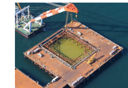
写真-5 大組・水中架設 Photo-5 Prefabricated panel placed by floating crane
