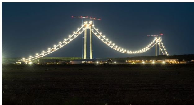
写真-5 吊橋全景 Photo-5 Bridge entire view
