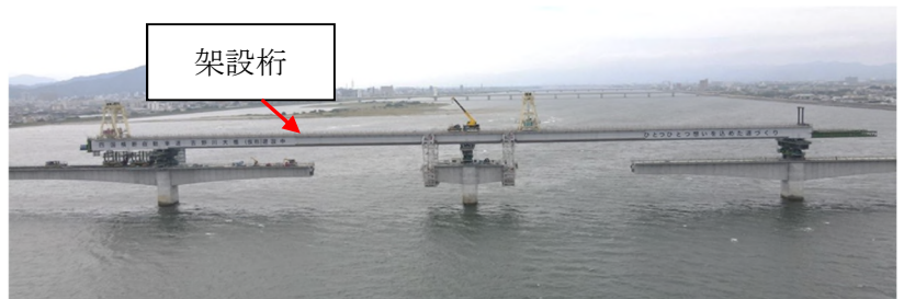
写真-4 架設桁架設状況 Photo-4 Erection girder
