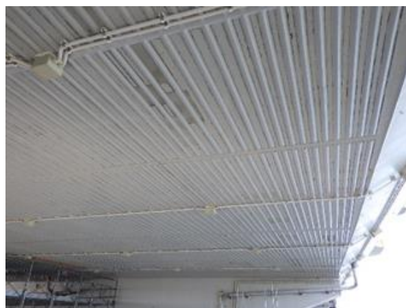
写真-2 回路設置完了 Photo-2 Cathodic protection equipment installed
