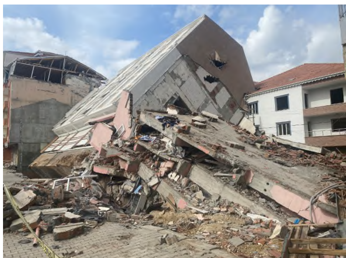
写真-4 崩壊した住宅建築 (Adiyaman) Photo 4 Collapsed Residential Buildings in Adiyaman
