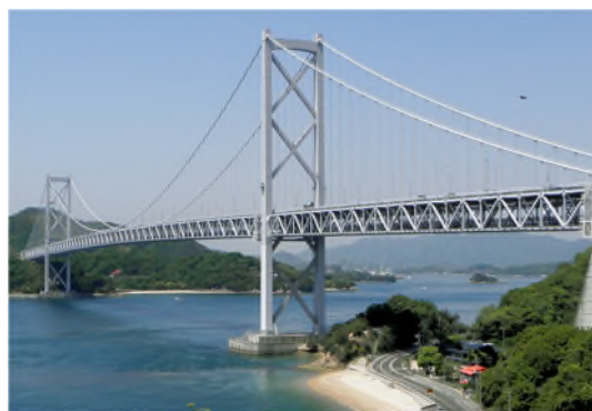
写真-1 因島大橋 Photo 1 Innoshima Bridge
