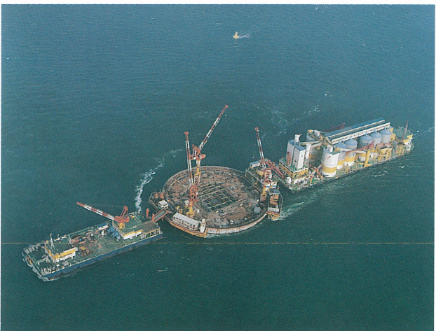
明石海峡大橋3P空撮
