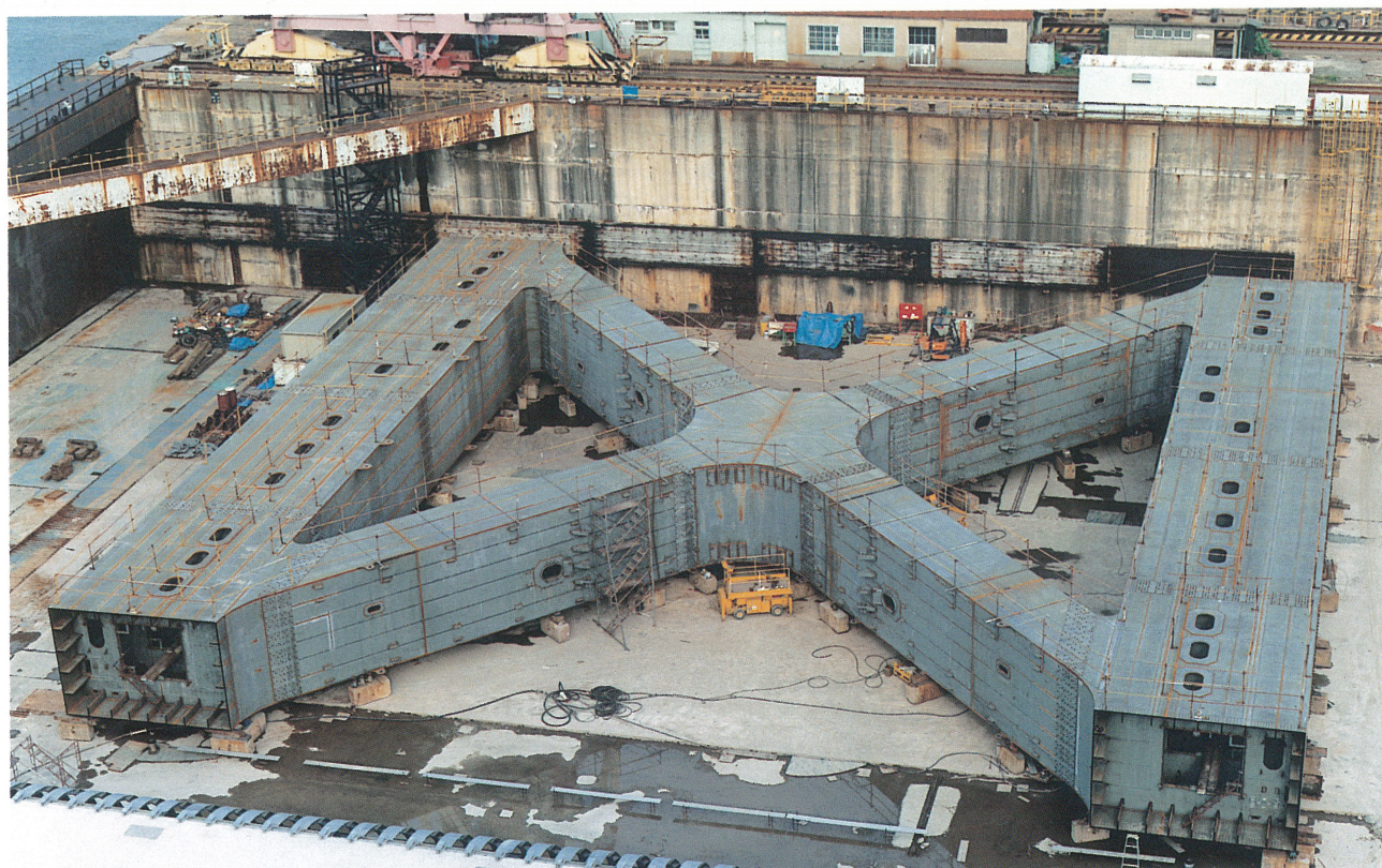
明石海峡大橋3P主塔工事 斜材仮組立 Shop assembly of the diagonal members , 3P tower
