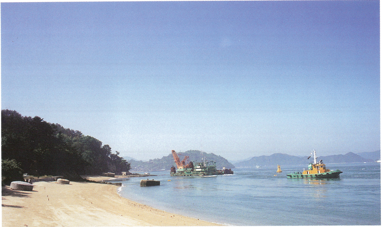
来島大橋下部工西工事 9P 海底掘削 Excavation of sea bottom for 3P 9P of the Kurushima Bridge
