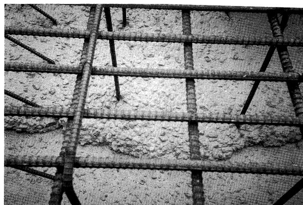
写真-3 L-10の流動先端 Photo.-3 Sence of flowing concrete
