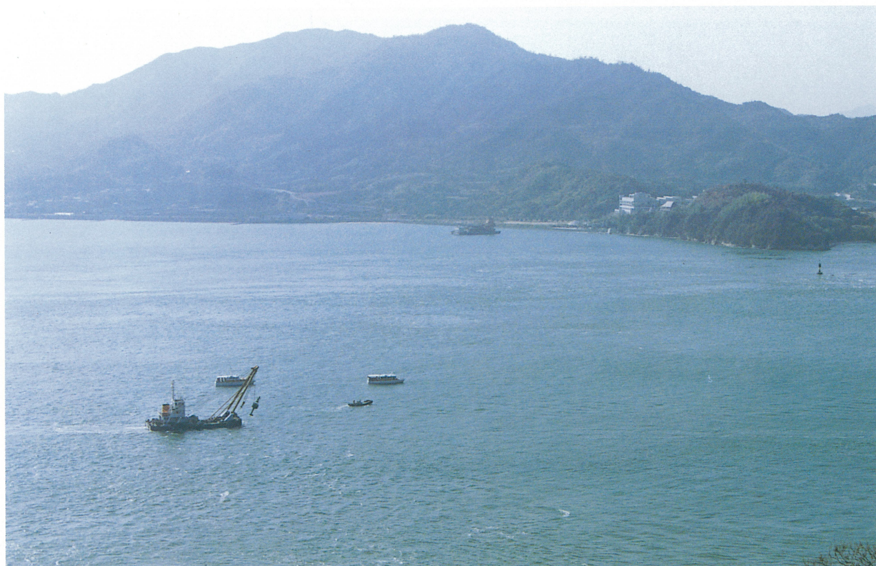
多々羅大橋2P灯浮標設置 Installation of lighting buoys to mark the work area for the Tatara Bridge 2P
