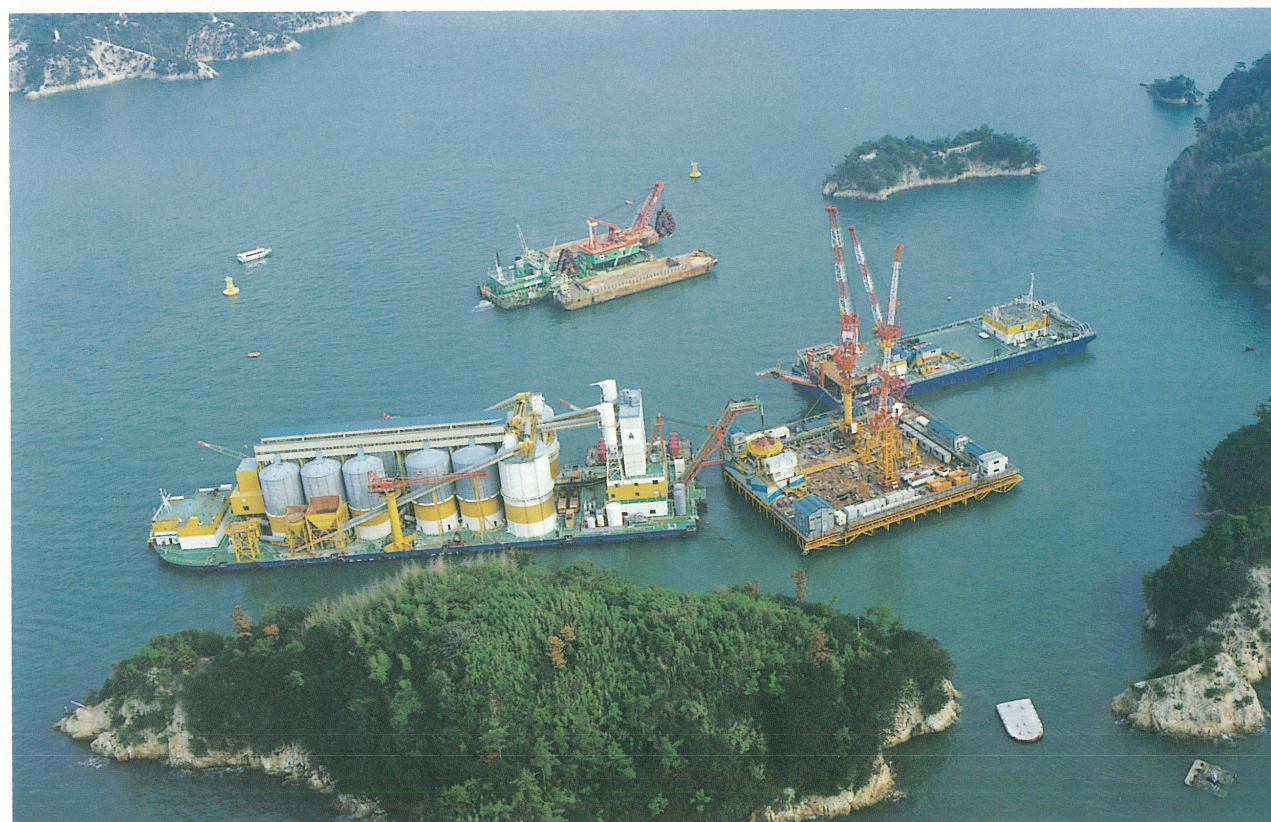
来島大橋4A 水中コンクリート工 (大型PC船の係留状況)、3P 海底掘削工 Mooring of a large-scale concrete plant barge used for underwater concreting for Kurushima Bridge 4A (front side), seabed dredging for 3P (back side)
