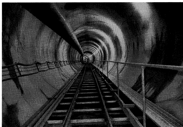
写真-3 導坑一般部 Photo.3 General section of pilot tunnel
