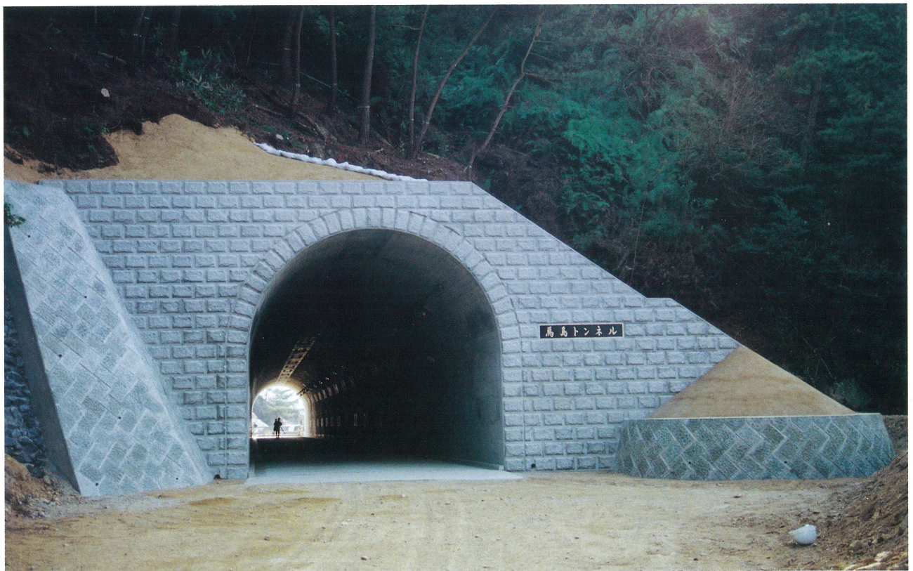
来島大橋 馬島々内付替えトンネル完成 Completion of a Relocated Tunnel in the Umashima Island
