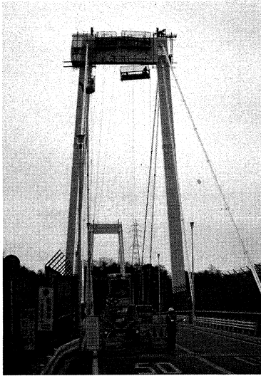
写真-5 2P 塔水平材足場 Photo.5 Scaffolding for lateral member of the tower 2P
