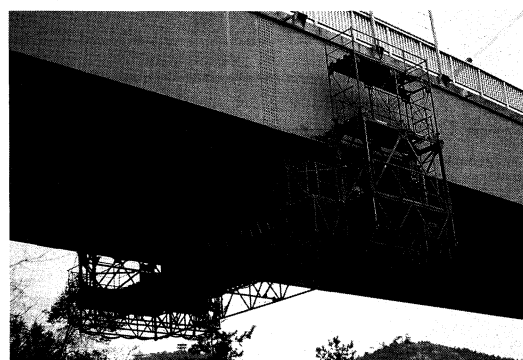
写真-16 移動式作業床 Photo.16 Movable work platform
