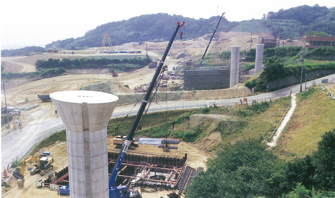
淡路IC(A.Fランプ橋)工事 Awaji IC (A.F Ranpe Bridge) Work
