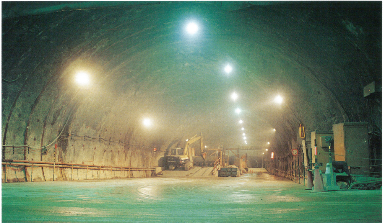
舞子トンネル工事現況(中南工事) The latest view of Maiko Tunnel work ( November 1993 )
