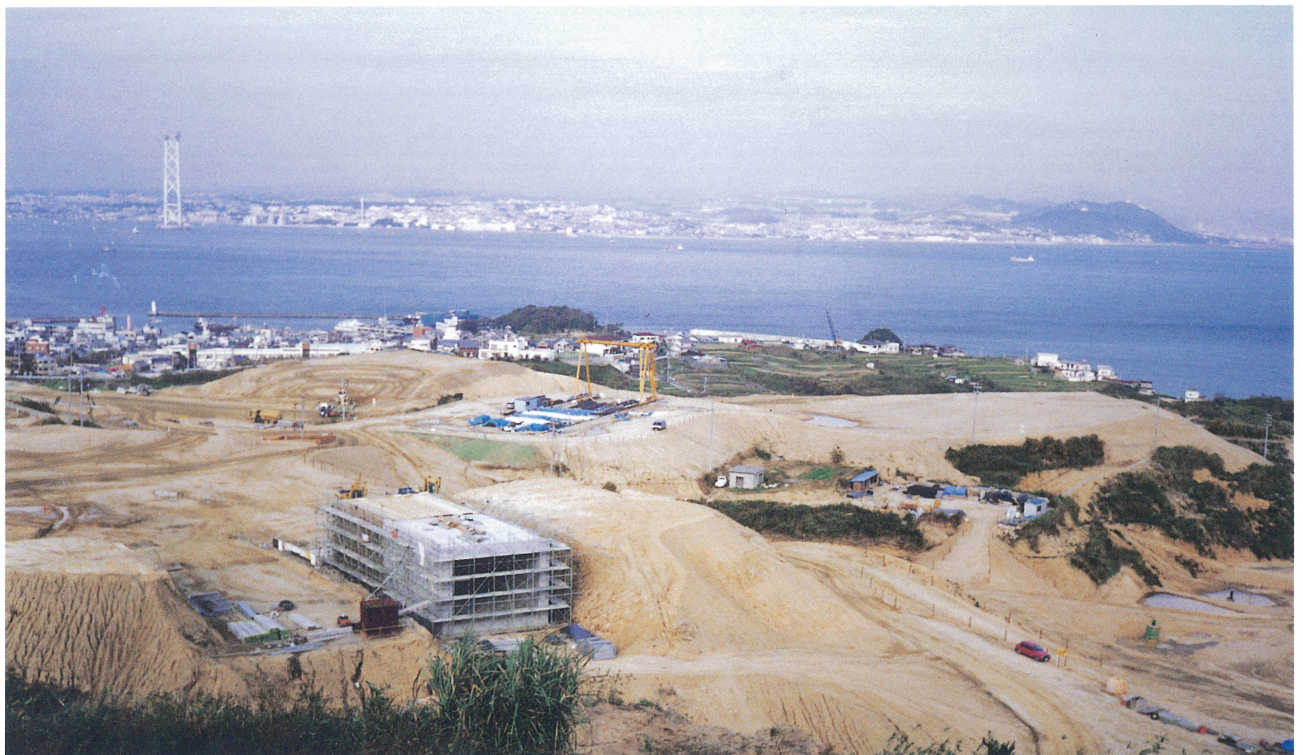
淡路ICの工事現況(「その1」工事) The latest view of Awaji Interchange work (Phase 1)(November 1993)
