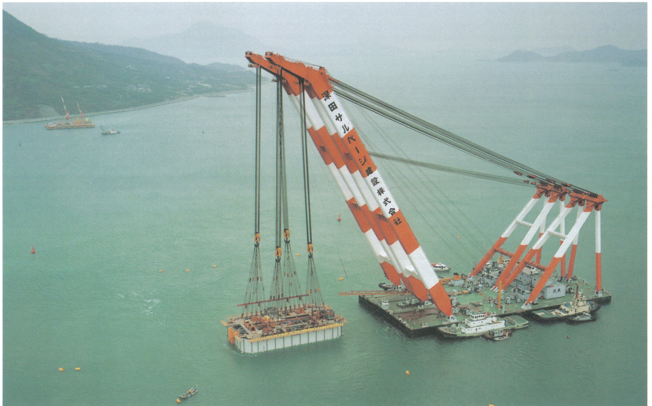
多々羅大橋3P鋼ケーソン沈設作業 Positioning work of Tatara Bridge 3P Steel Caisson (December 21, 1993)
