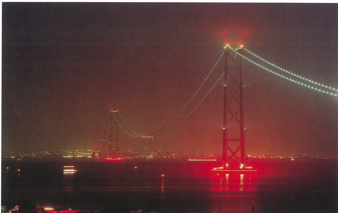
夜間照明の明石海峡大橋 Akashi Kaikyo Bridge illuminated by work lights
