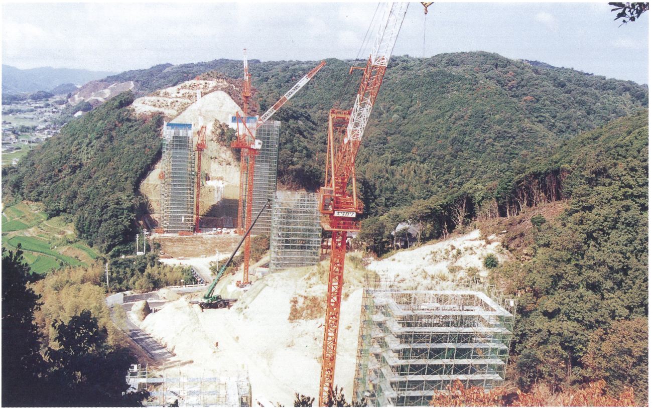
楠本川橋工事 Work of Kusumoto-gawa Bridge
