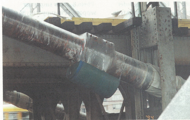
写真-4 注入された油を回収 入出量で注入量管理 Photo.4 Removal work of poured oil-Residual quantity is checked by in and out quantity.
