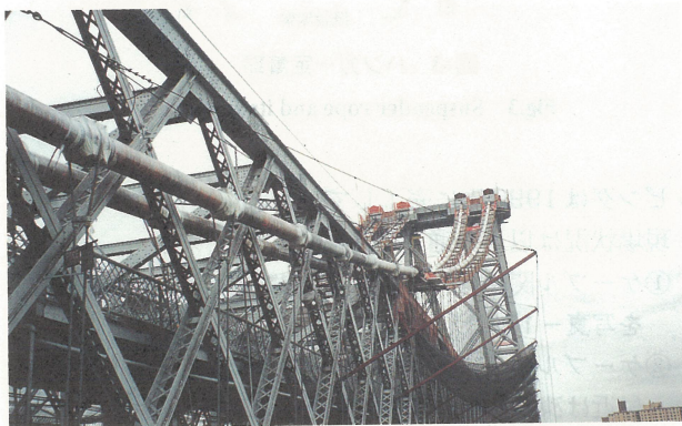
写真-3 ケーブルは油注入のため、補修後ビニール被覆 Photo.3 Cable is wrapped in vinyl to prepare for pouring oil after repairs.
