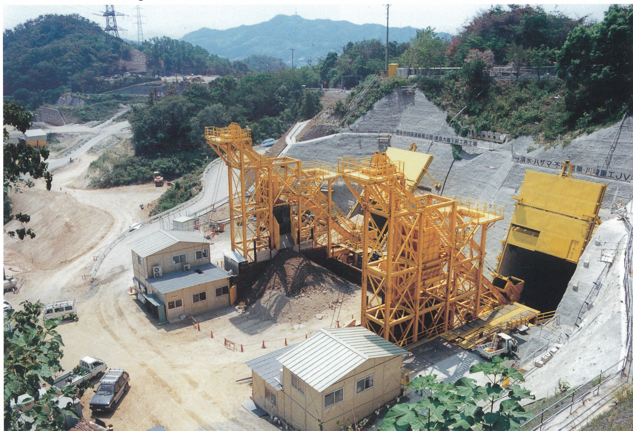
来島大橋 10A 南北斜坑設備 Work Equipment in North & South Inclined Shafts for Kurushima Bridge 10A
