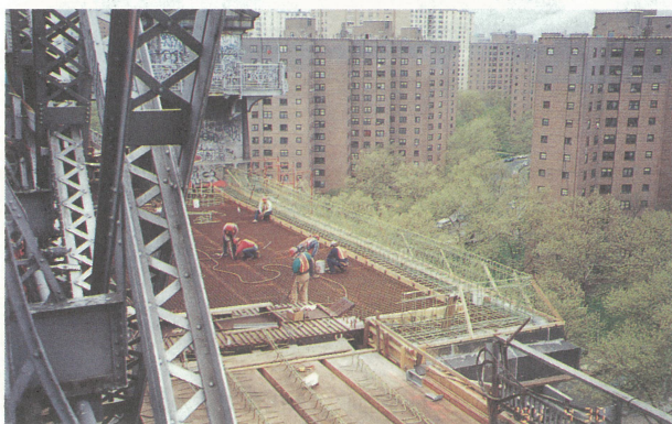
写真-9 アンカレイジ部床版補修 I型格子床版・塗装鉄筋使用 Photo.9 Repairs of floor slab—I-beam grid and coated rebar were used.
