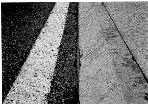
写真-2 完了状況 Photo.2 Finished view of work
