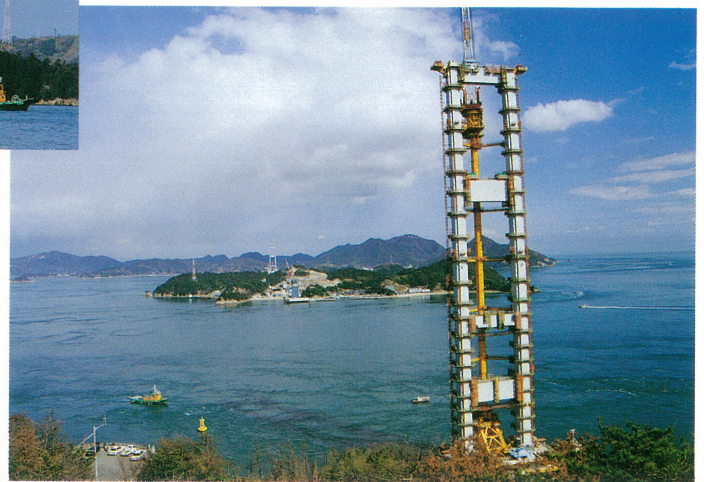
来島大橋(手前は9P主塔、向こうは馬島) (7年3月) Kurushima Bridge (front side : 9P Tower, back side : Umashima Island) March 1995
