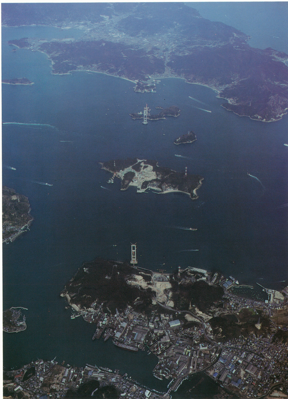
来島大橋の工事現況 Current view of Kurushima Bridge work
