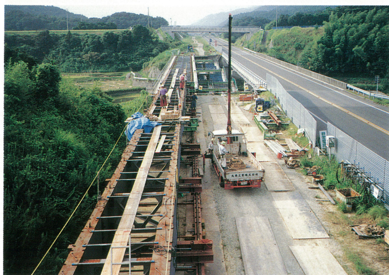
津名皿池橋鋼上部工工事 [淡路島内四車線化区間] Tsuna-saraike Bridge superstructure work for 4-lane widening part in Awajishima island
