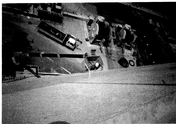
写真-5 目地シール施工条況 Photo.5 Sealing of joint
