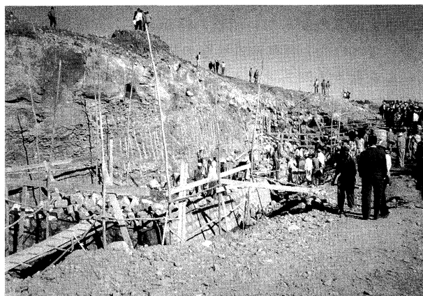
写真-2 建設中の下部工（石積工が多い） Photo.2 Substructure under construction (Masonry structure is mostly employed.)
