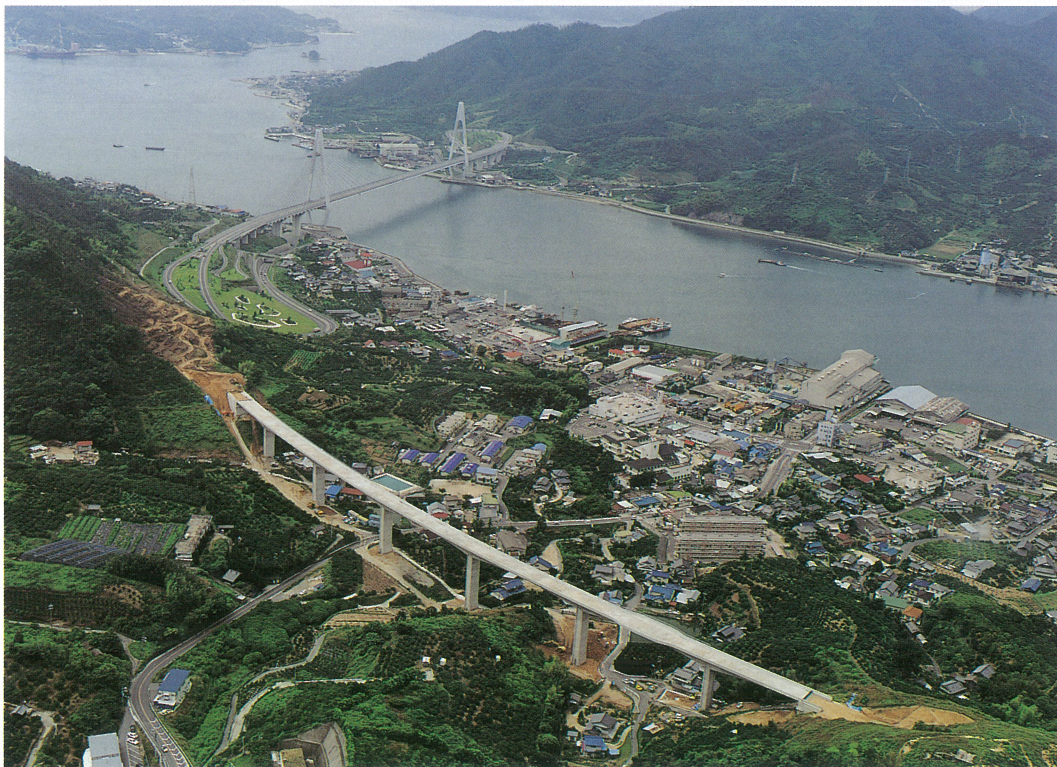
西浦高架橋の完成、上空より望む Completion of Nishiura Viaduct, Bird's-eye view
