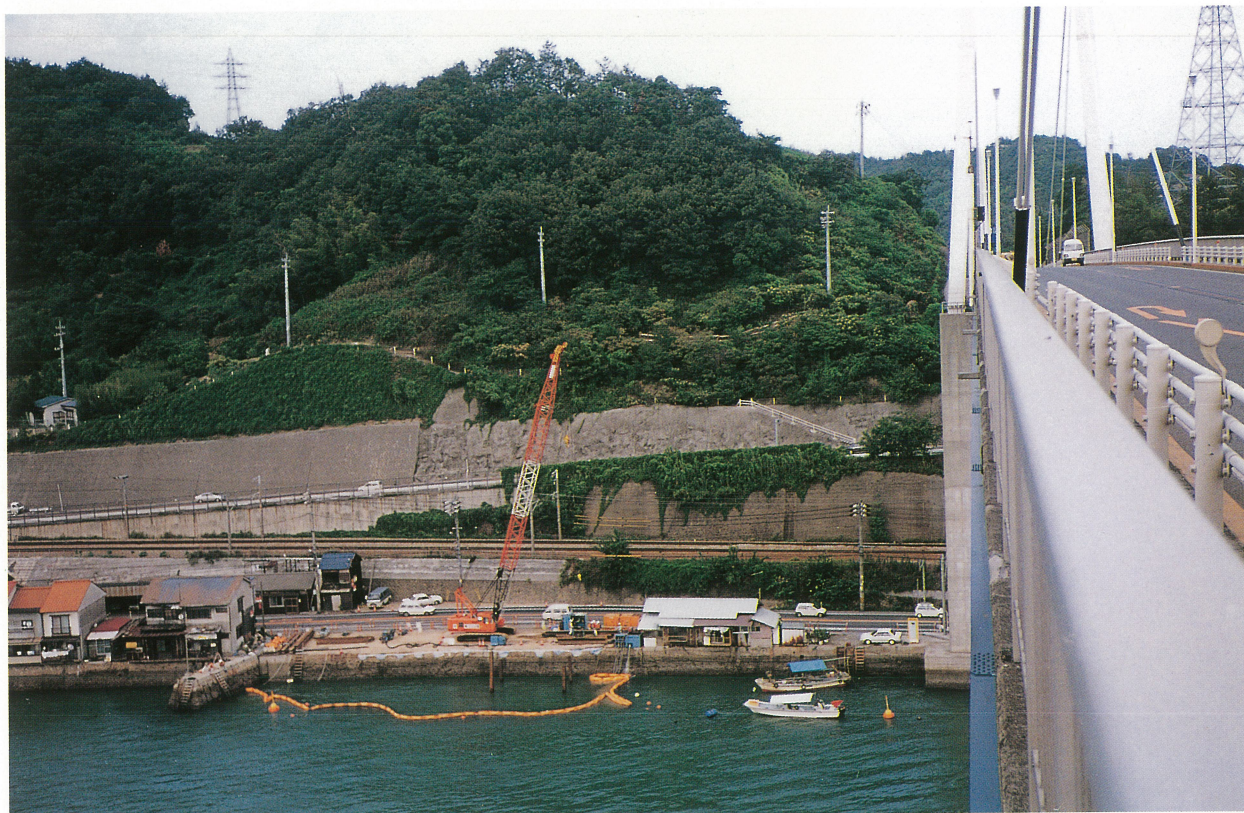
新尾道大橋 2 P [灯浮標の設置] Shin Onomichi Bridge 2P--Installation of lighting buoys
