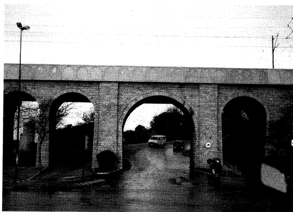
写真-10 ラバト近郊サレの鉄道高架橋 Photo.10 Railway viaduct at Sale near Rabat
