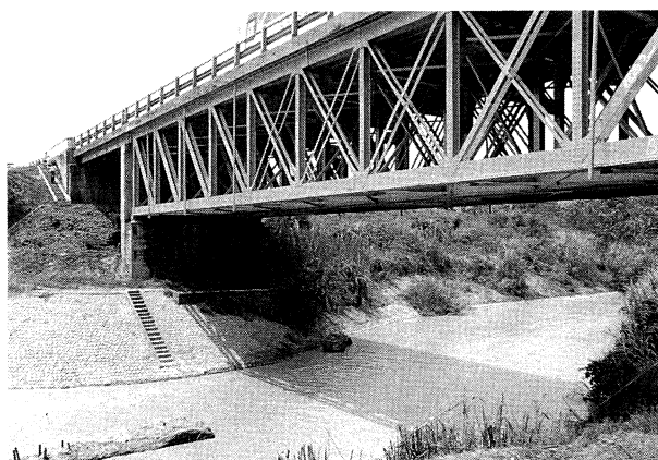
写真-2 CILAMAYA 橋 Photo.2 Cilamaya Bridge
