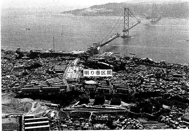
写真-1 明り巻区間全景 Photo.1 Overview of open-cut portion
