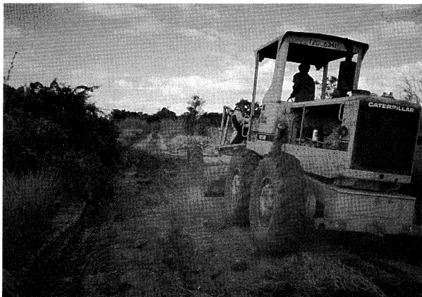
写真-2 道路補修状況 Photo.2 Road repair work
