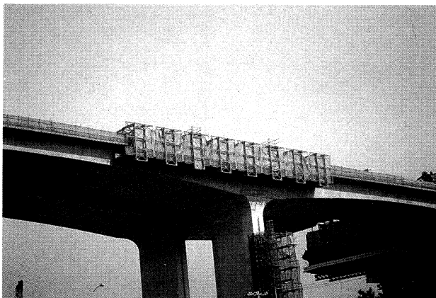
写真-6 防護作業台車(P6) Photo.6 Work vehicle for safety apparatus
