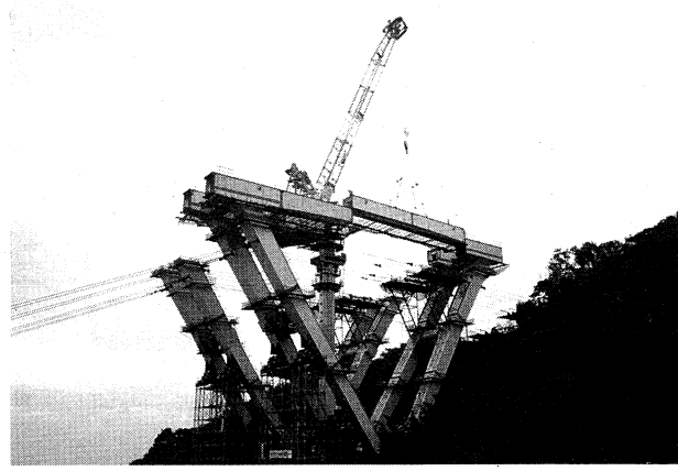
写真-3 P7の架設状況(V脚中央落とし込み) Photo.3 Construction of P7 (settlement of V pier in center)
