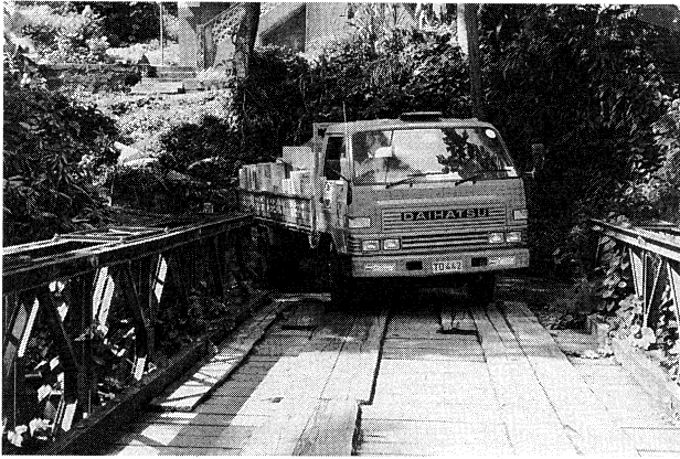
写真-5 橋梁の状況 Photo.5 Condition of bridge
