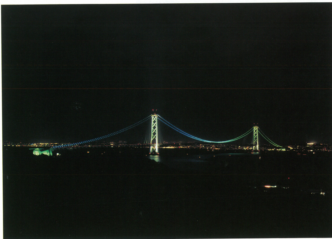
試験点灯中の明石海峡大橋 General view of Akashi-Kaikyo Bridge on lighting test
