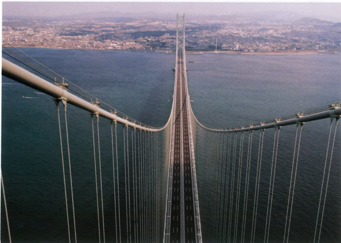
舗装完了 Completion of pavement
