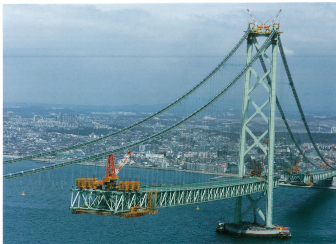
補剛桁架設 Erection of stiffening girder
