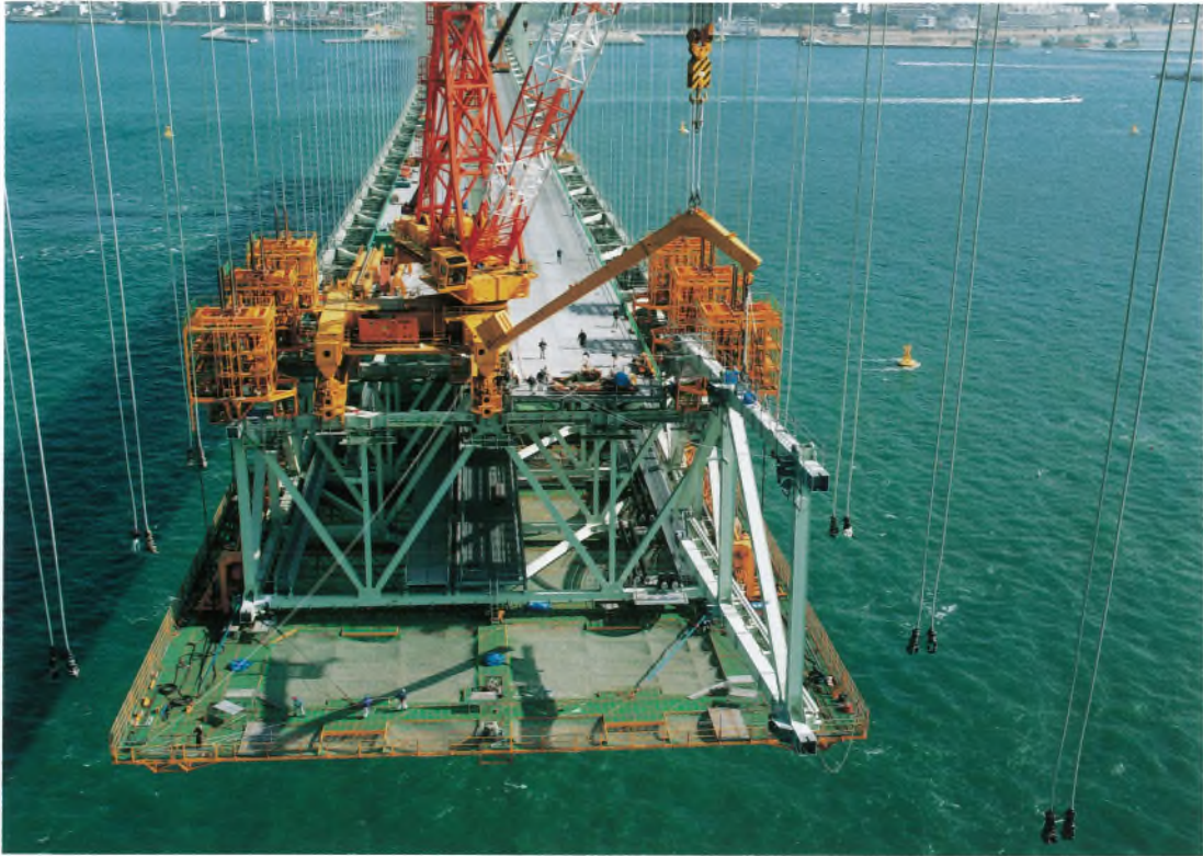
補剛桁架設 Erection of stiffening girder
