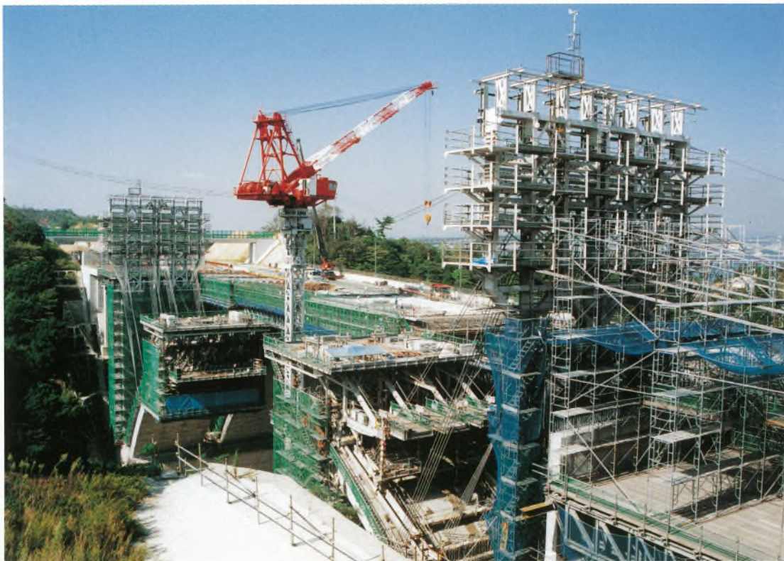
茶間川橋 Chamagawa Bridge
