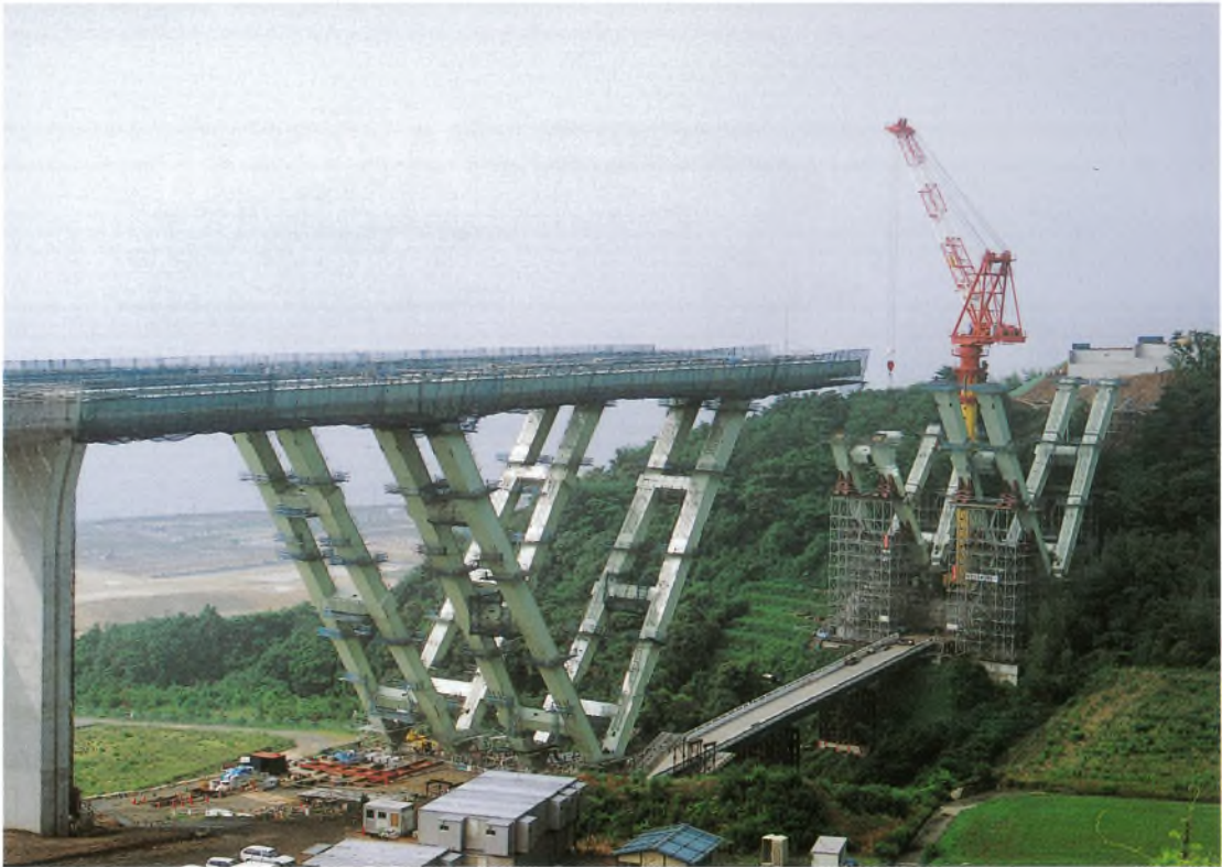
灘川橋 Nadagawa Bridge
