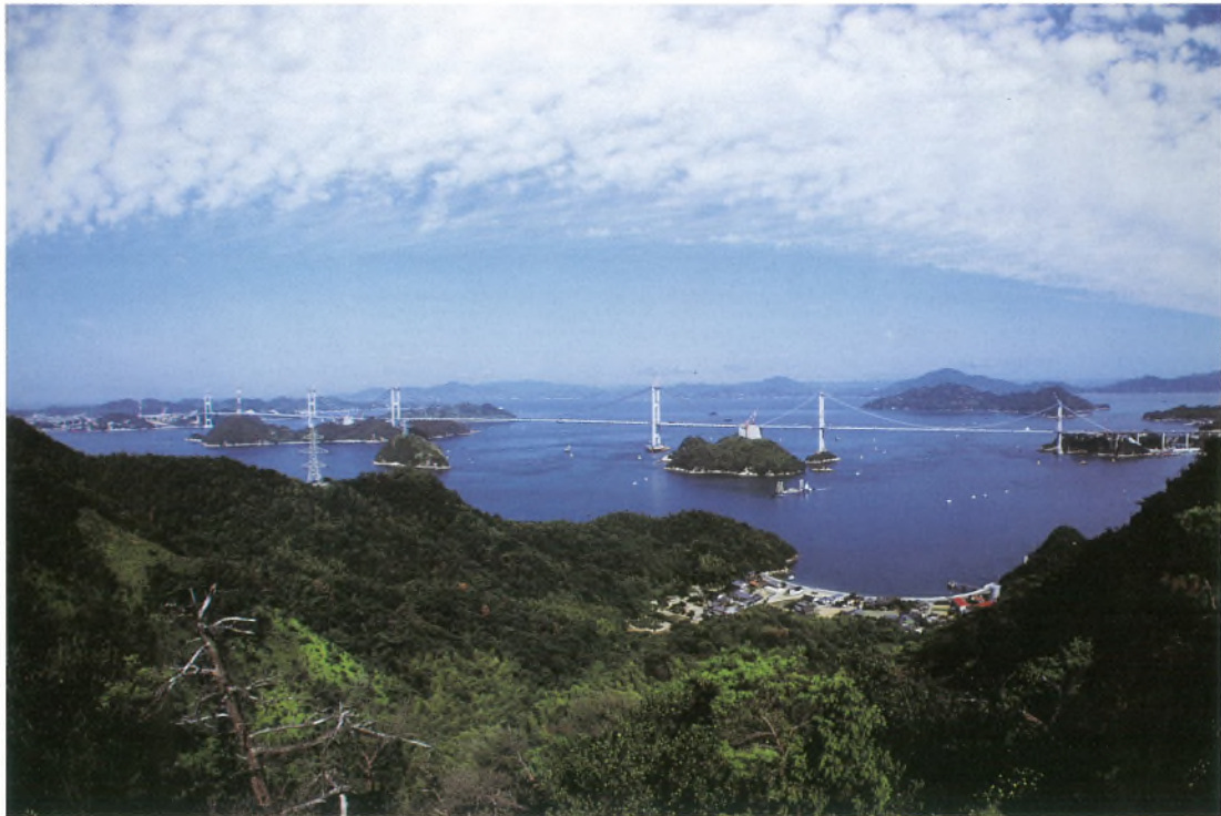
来島大橋工事現況 Current view of Kurushima Bridge work
