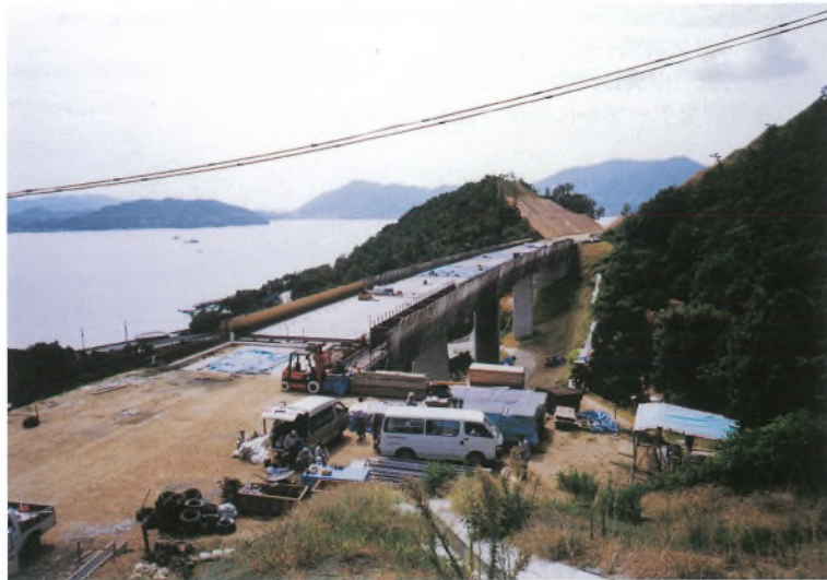
天神川橋工事現況 Current view of Tenjingawa Bridge work
