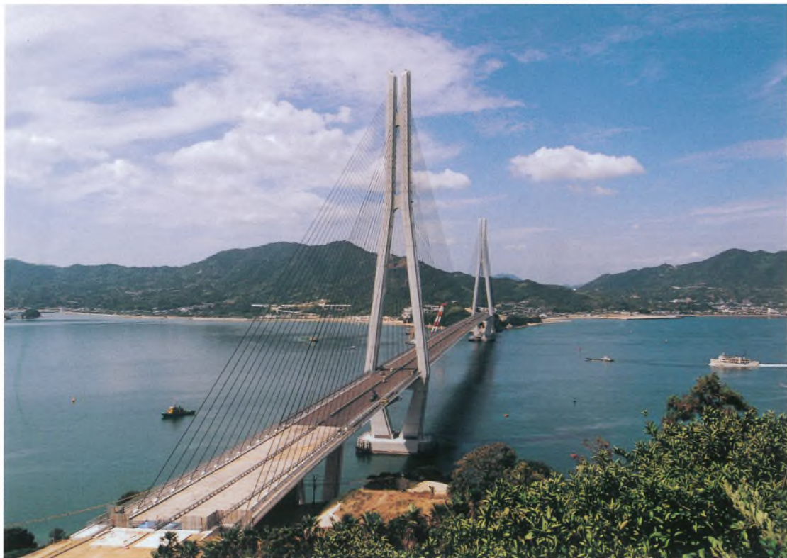
多々羅大橋工事状況 Current view of Tatara Bridge work
