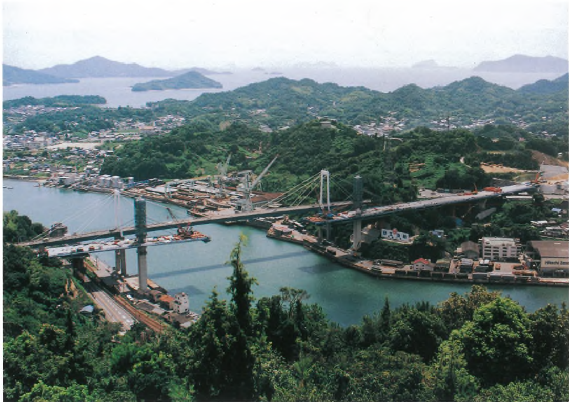
新尾道大橋工事現況 Current view of Shin Onomichi Bridge work
