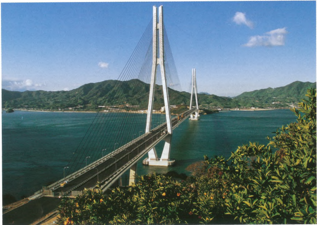
多々羅大橋工事現況 Current view of Tatara Bridge
