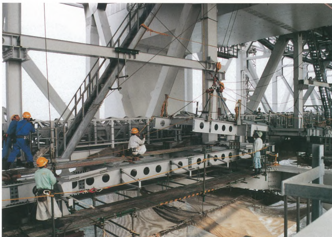
4 P 部付近連絡通路主桁架設状況 Girder installation near 4 P
