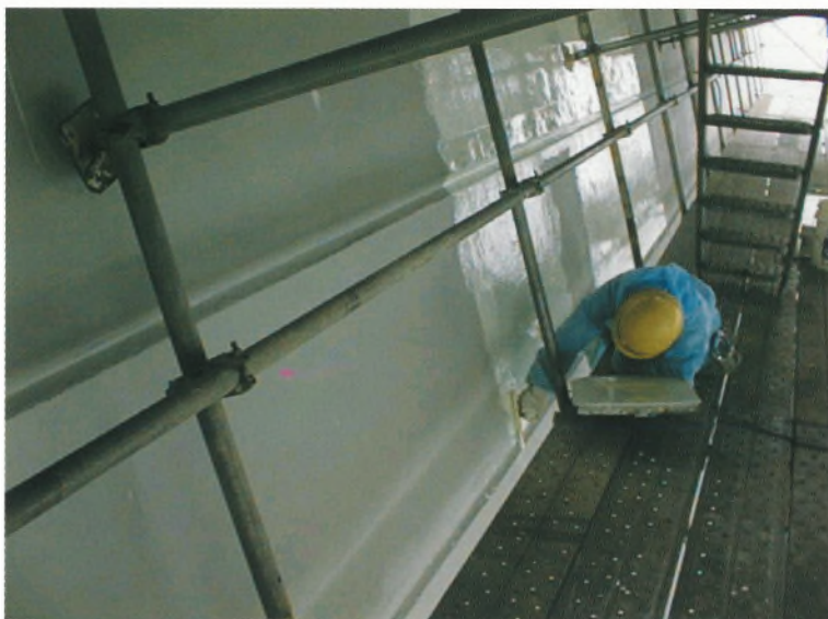
中塗り作業状況 Work on secondary coating
